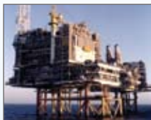
1995 – Eastern Trough Area Project, BP, North Sea
