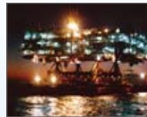
1995 – Wandoo Oil Field Development, Ampolex Limited, Australia
