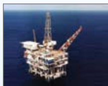
1983 – Lena Guyed Tower, Exxon, Gulf of Mexico
