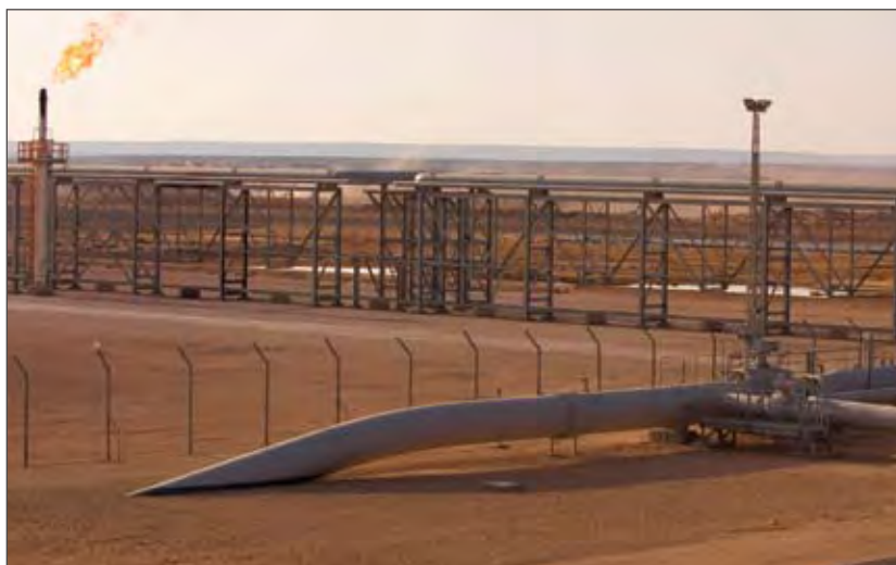
Delivering the FEED and full EPC of the world's first full-scale carbon dioxide capture project at a gas field, KBR and its joint venture partners are helping the environment by making it possible to inject about one million tons of CO 2 into a reservoir each year.
