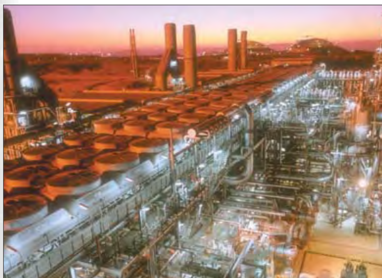
Trains 1 & 2 of Woodside's North West Shelf LNG's production facility hailed as the world's first fully air-cooled liquefaction plant.
