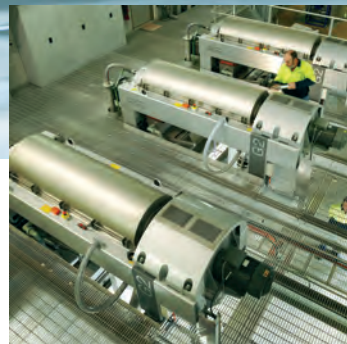
Christies Beach plant upgrade, South Australia
