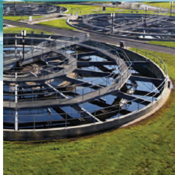
Upgrade of tertiary treatment, Eastern Treatment Plant, Victoria
