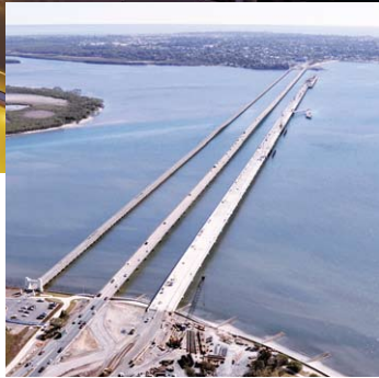
Houghton Highway duplication, Queensland
