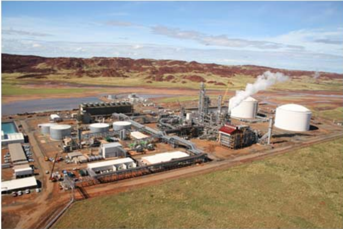
Figure 2 Overview of BFPL Complex
