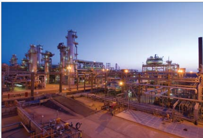
BP turned to KBR and its joint venture for full EPC services, infrastructure and construction management for the largest dry gas project in Algeria – In Salah.
