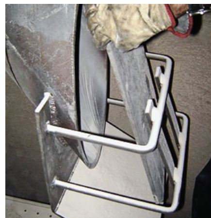
FIG. 7 Cyclone dipleg check valve.
